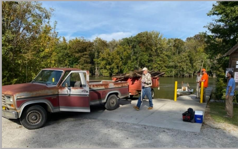
Out with the OLD: Hauling away the old decking.
